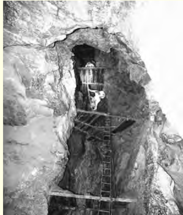
Figure 3. Wooden staircase in Grotta di Trebiciano, Trieste, Italy. These staircases have been initially installed in 1894 during the investigation for providing water for Trieste. The platforms (top in the photo) were installed one century ago in pitchpine treated with copper sulfate and carbonileo (Photo Maizan/SAS).
