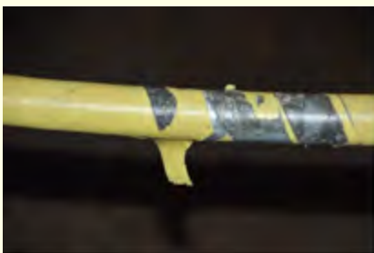
Photo of damaged yellow tape on a handrail that needs repair.
