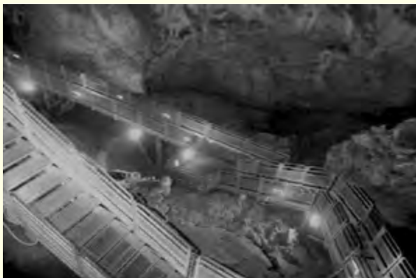
Figure 2. Zinc plated iron pathways in the Su Mannau Cave, Sardinia, Italy (Photo Cigna).
