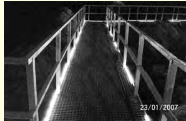
Figure 4. The emergency lights placed along the edge of the pathway in the Grutas de Bustamante, Mexico (Photo Cigna).
